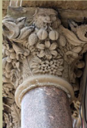
Palantine Building, Prince William Street
